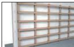
Horizontal battens on top of vertical battening = installation CSP vertical.
