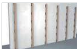
Only vertical support battening = installation CSP horizontal.
